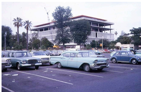
Construction of the Gordon D. Schaber Courthouse, circa 1963
