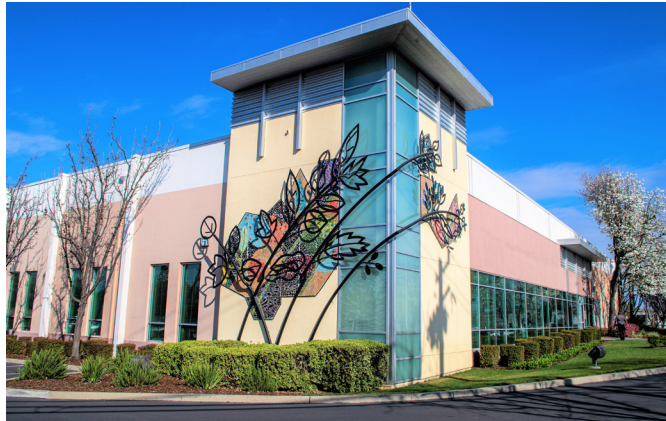
SETA Office, 925 Del Paso Blvd.
